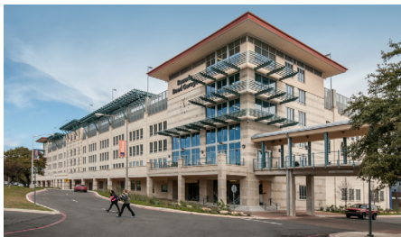
The University of Texas at San Antonio, Bauerle Road Parking Garage; $31,673,537; 425,000 SF; San Antonio, TX
