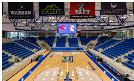
Northside ISD, Northside Sports Gymnasium; $26,632,762; 88,000 SF; San Antonio, TX
