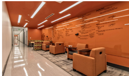
UT Health San Antonio, Facility Renewal & Renovation School of Nursing & Dental School; $36,607,079; 167,550 SF; San Antonio, TX
