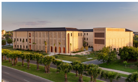
The University of Texas Rio Grande Valley, Academic Building; $38,132,500; 124,000 SF; Brownsville, TX
